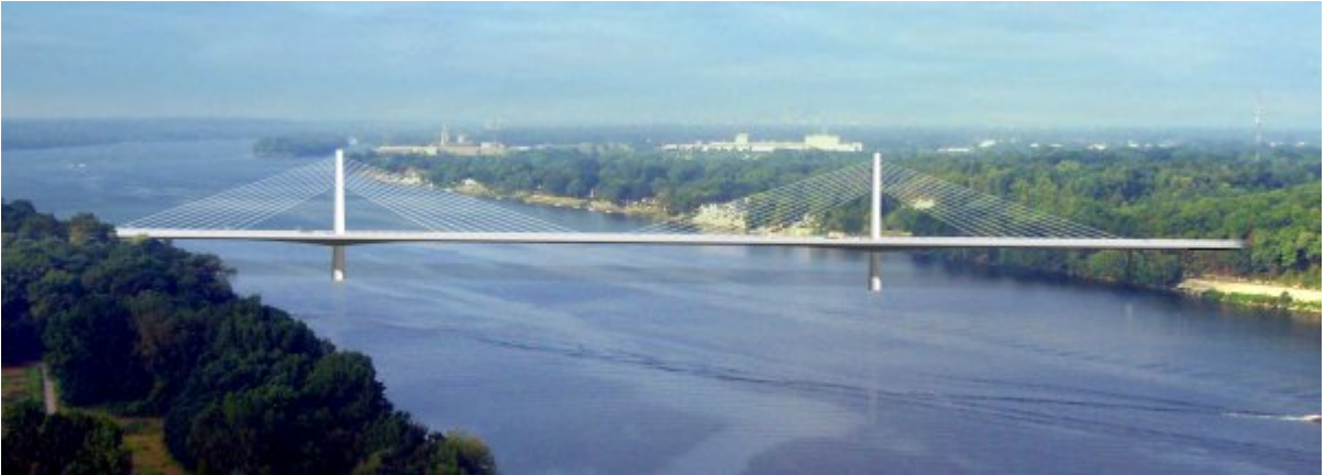
A5 Aerial View
