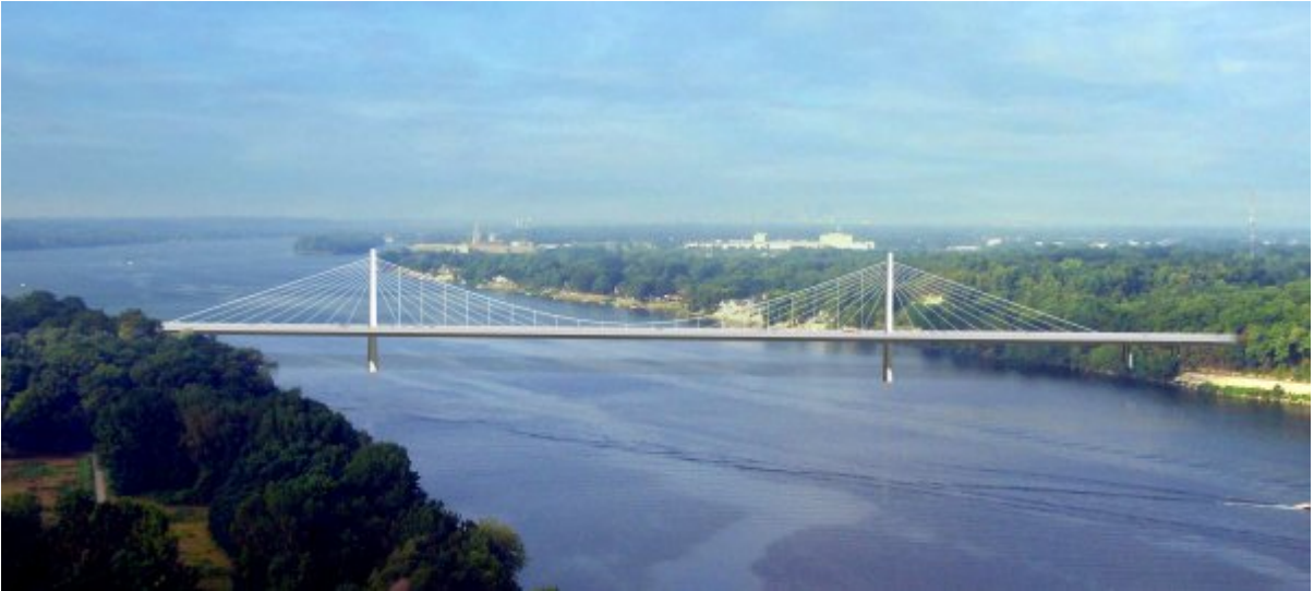
A6 Aerial View
