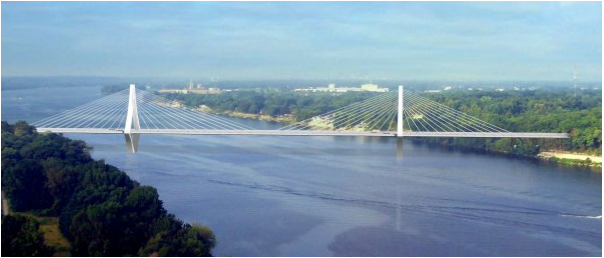
A2 Aerial View
