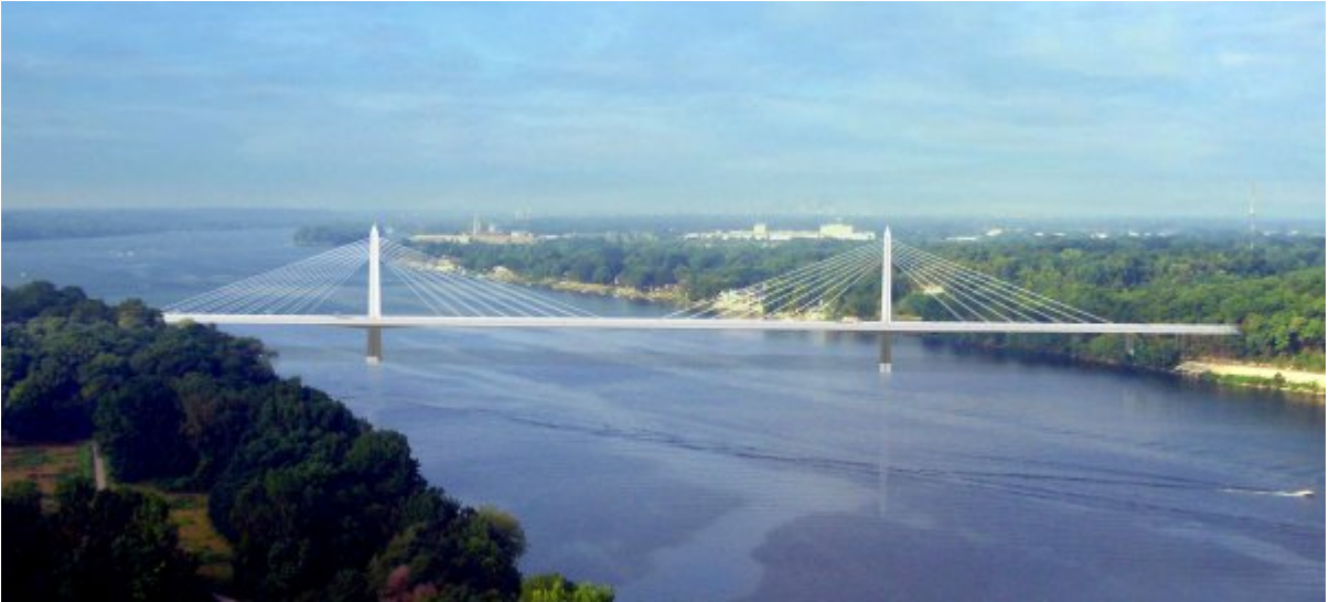
A4 Aerial View
