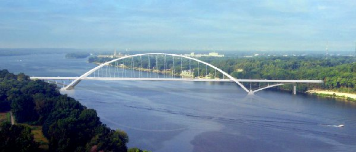
A1 Aerial View
