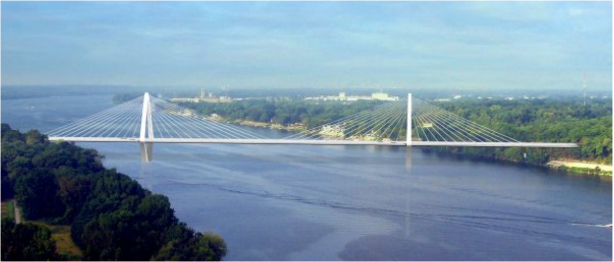
A3 Aerial View
