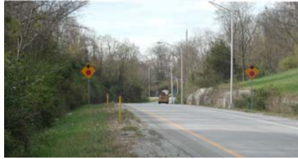
Roadway view showing US 42 northbound exit ramp to half diamond interchange
