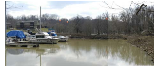
View from marina parking lot in The Harbor at Harrod's Creek and renderings
