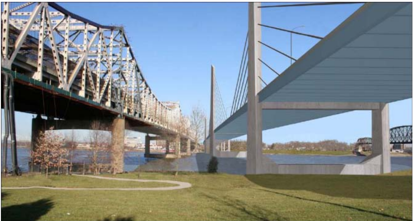
ALTERNATIVE 2 – LOOKING TOWARD INDIANA BETWEEN BRIDGES
