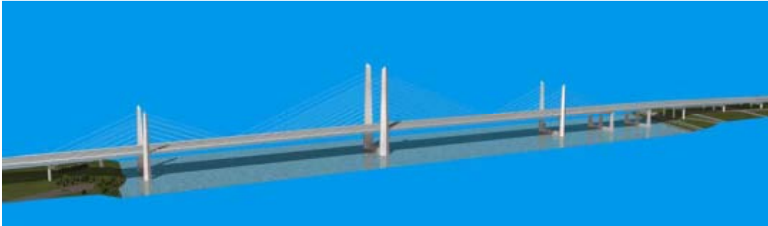
Alternative 2: Three Tower Cable-Stayed
