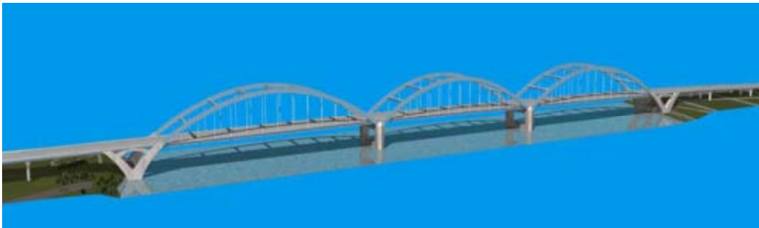
Alternative 3: Three Span Thru Arch
